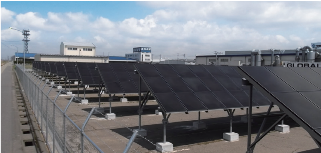
Utilizing renewable energy in its business operations, Twinbird installed solar power generation systems on the premises of its Head Office, with their maximum output totaling 250kW.
